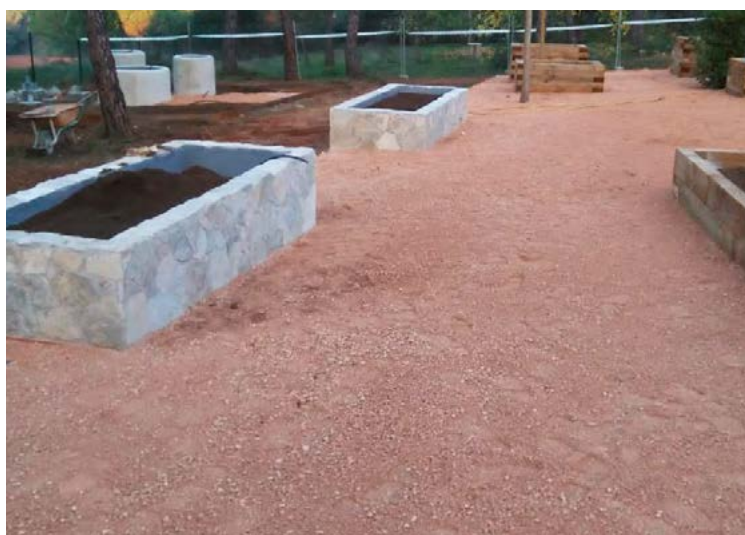
Image 28. Decomposed granite must be packed very well if to be used by wheelchairs. Photo JTP
